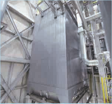
Filtration-type dust collector This system uses rows of tubular filters to filter exhaust gas treated with slaked lime and activated carbon, removing harmful substances such as sulfur oxides and hydrogen chloride as well as dust.
