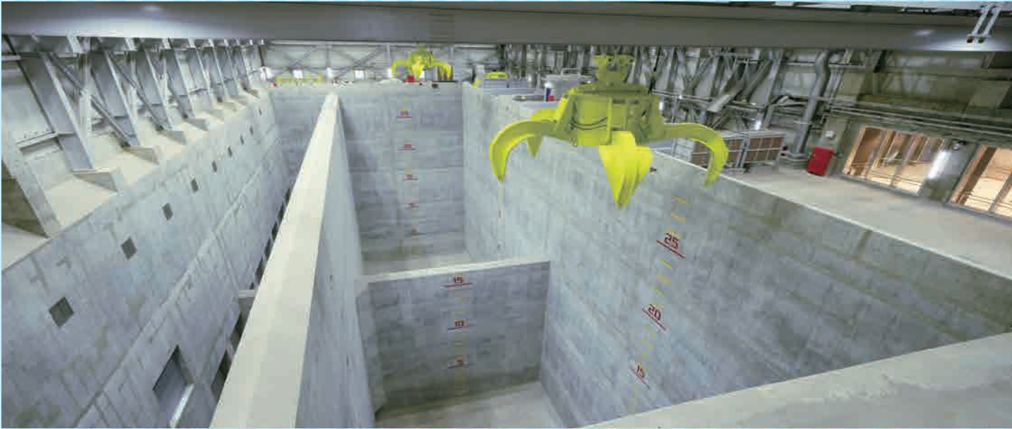
Waste pit Waste dumped into the receiving pit is transferred by waste crane into the stirring pit, where it is stirred so that it burns well. The capacity of the waste pit is 26,000 m 3 (equivalent to about fifty 25-meter swimming pools).
