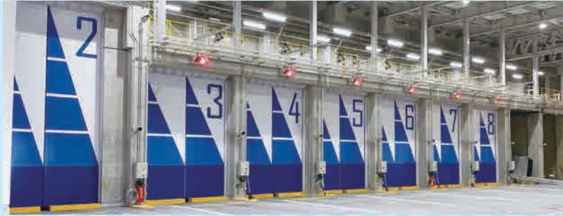
Platform After the garbage trucks are weighed, they dump their contents into the waste pit through one of eight loading gates. A double gate system and controlled air pressure are employed to prevent odors from leaking out.
