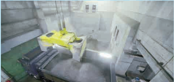
Ash pit and fly ash processing pit Incinerator bottom ash, generated from burning waste in the incinerator, and the fly ash collected from the boiler and filtration-type dust collector are stored here.
