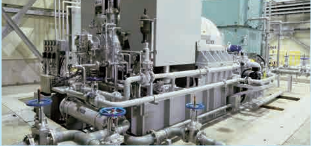
Steam turbine generator High-temperature, high-pressure steam sent from the boiler turns turbines to generate power from waste with high efficiency.
