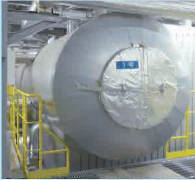
Boiler Heat from the exhaust gas produced from incinerating waste is used to generate high-temperature, high-pressure steam, which is then sent to the turbine.
