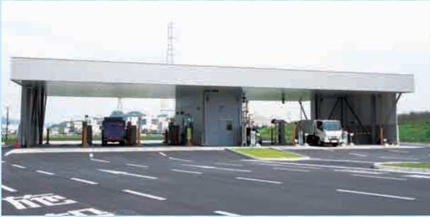
Truck scale Each vehicle is weighed on a truck scale to total the amount of waste collected.
