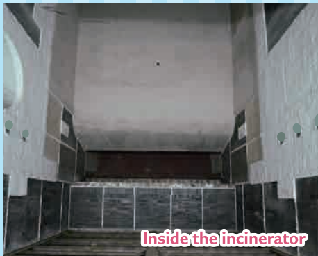
Incinerator Combustion in the incinerator is controlled automatically to burn waste completely. The combustion takes place at temperatures over 850°C to reduce the production of harmful substances, including dioxins. High-temperature air combustion technology enables stable combustion using less air for greater energy efficiency.
