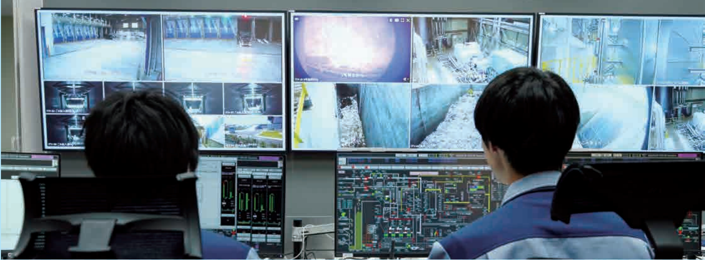
Central control room From this room, the operational status of the entire facility is monitored (including the temperature inside the incinerator and the concentration of harmful substances in the exhaust gas) and equipment is operated remotely. Remote monitoring and remote operation from outside the facility is also used to ensure the safe, stable treatment of waste.
